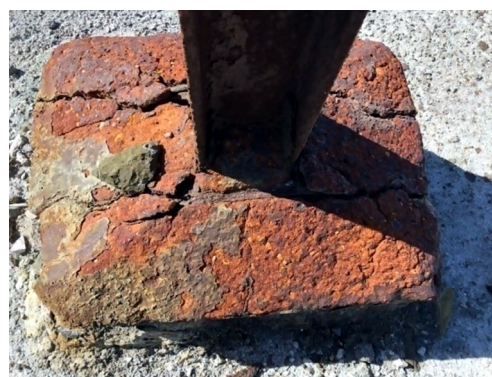
Fig. 8 Concrete support and metal mine beam affected by acidic water
